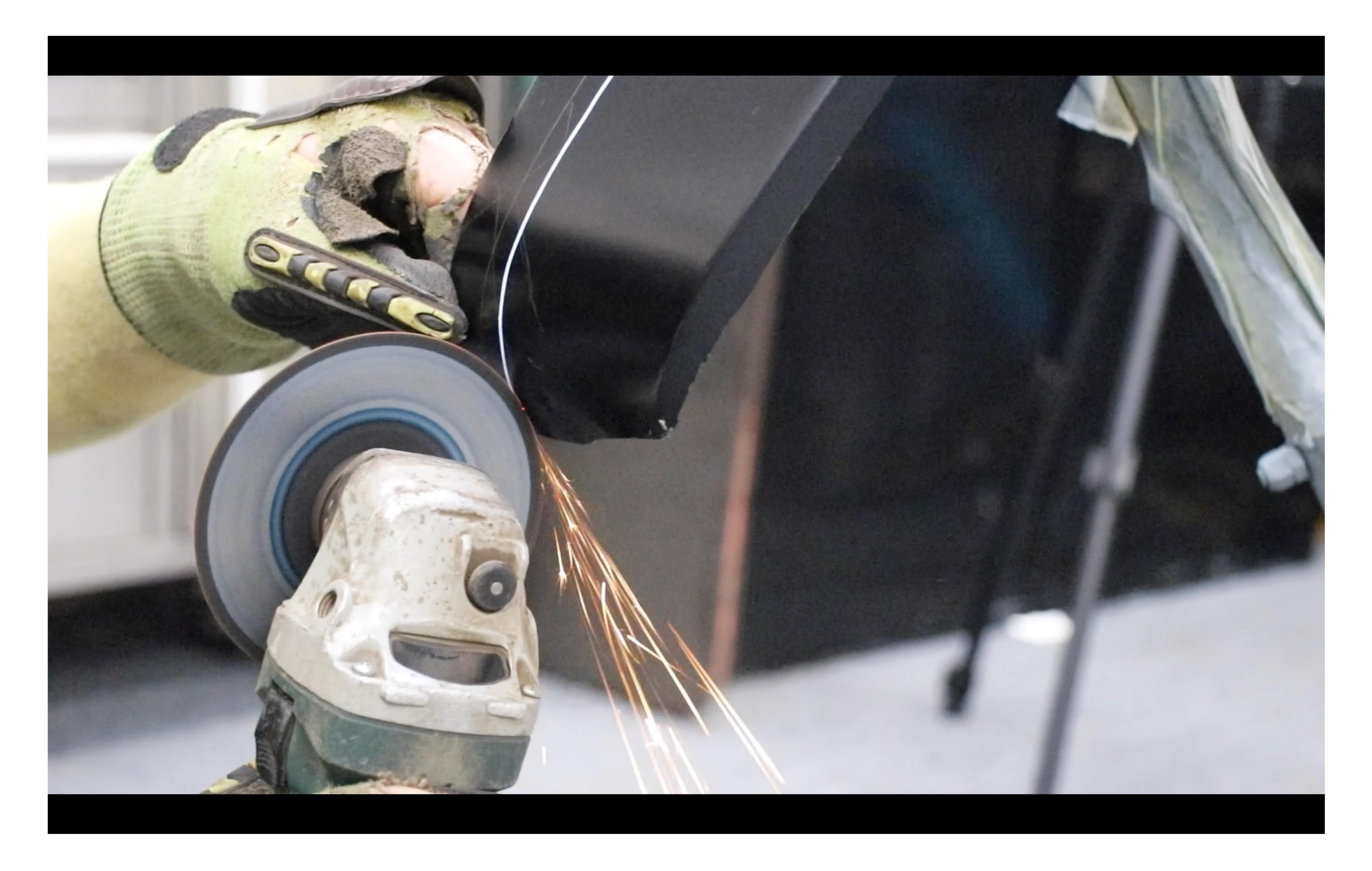
Now cut inside line using appropriate cutting tool, and correct PPE.
